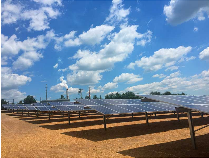
LG&E/KU E.W. Brown Generating Station: 10 MW
